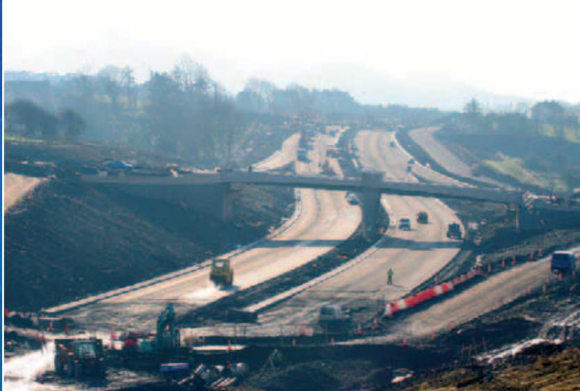
Sligo inner relief road under construction
