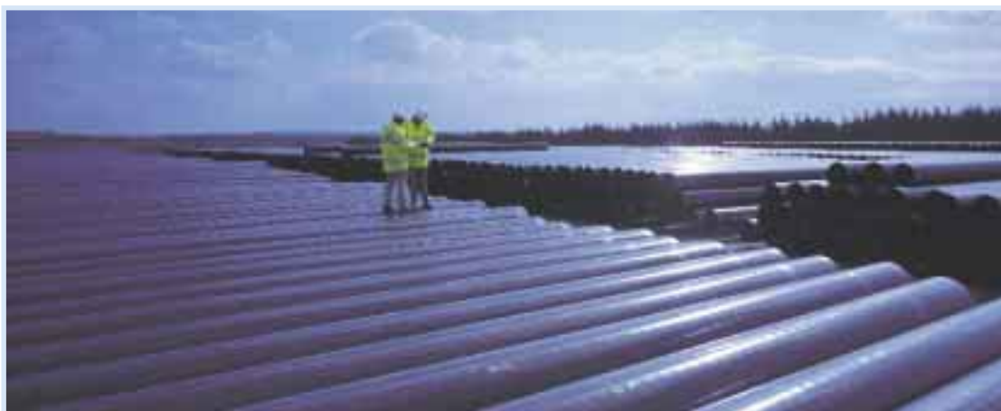
Gas pipe storage
